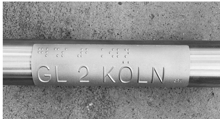
Figure 2. Handrail Printed with Braille for Visually Impaired People
